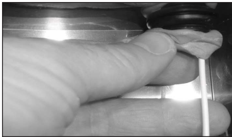
10. Close the inside hole by using putty
