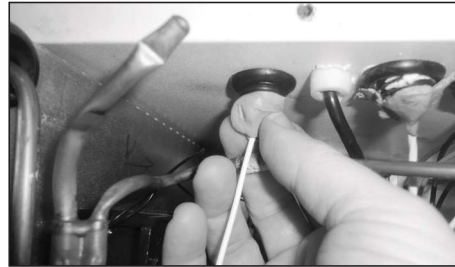
9. Closed the port hole by using putty
